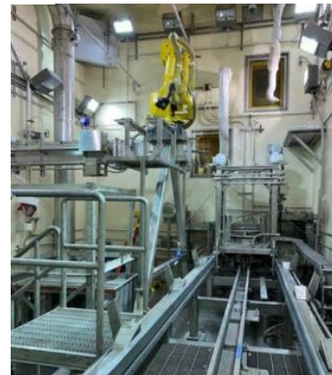
Progress toward start-up of Integrated Waste Treatment Facility
