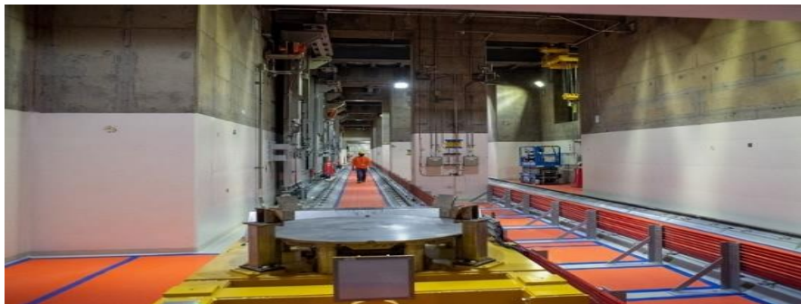
Construction completed at Low-Activity Waste Facility (vitrification)
