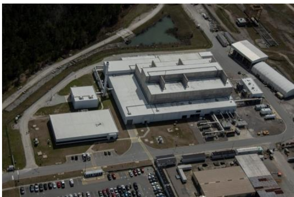
Hot Commissioning of Salt Waste Processing Facility
