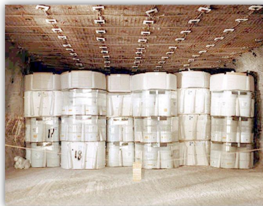
Drums of transuranic waste in specially mined disposal panels underground at WIPP Source: U.S. Department of Energy
