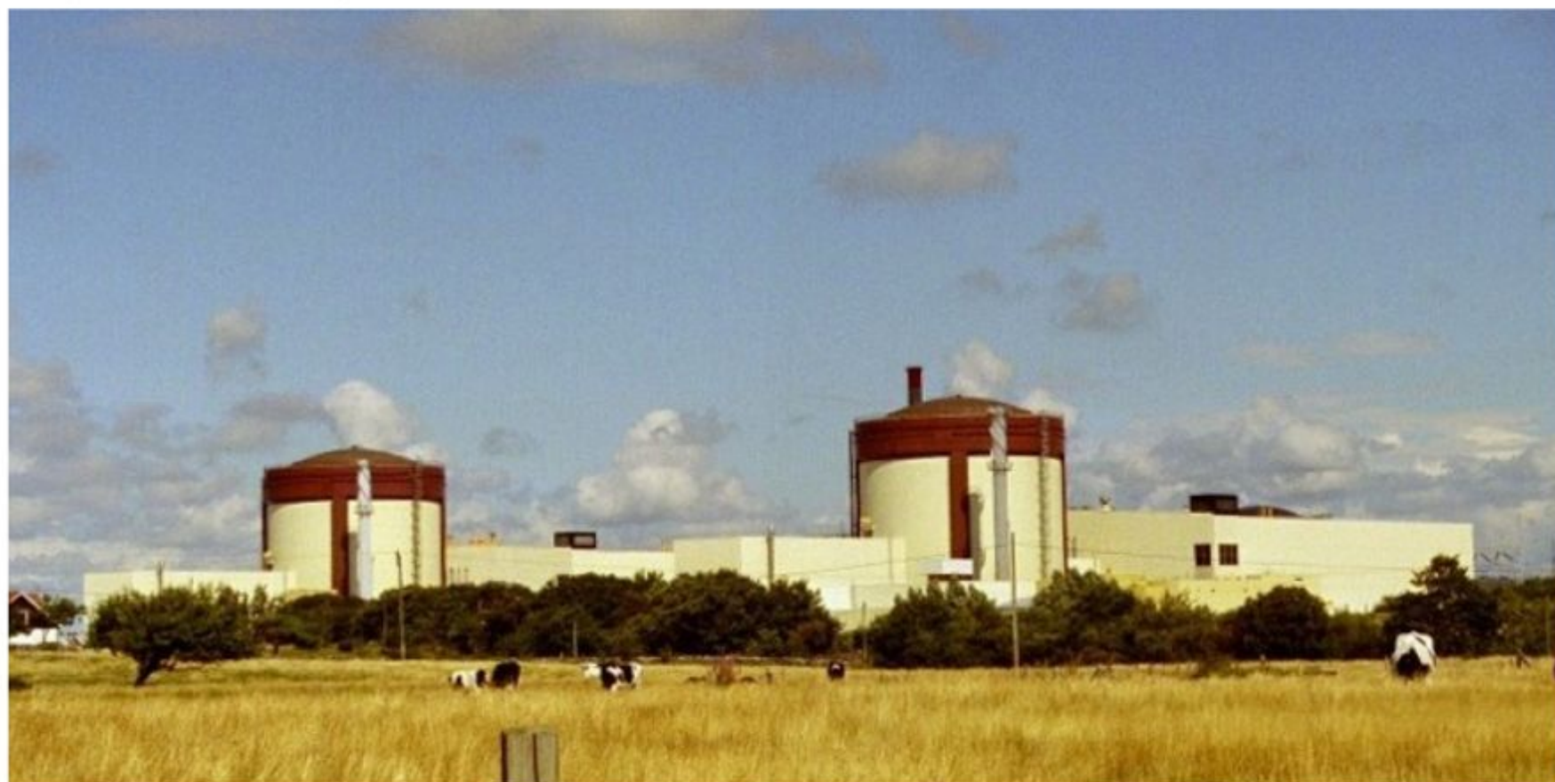
The Ringhals nuclear power plant. (Photo: Wikipedia)
